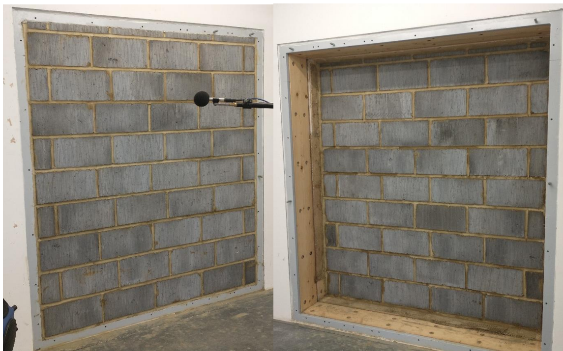
Figure 4.1- Photograph images of breezeblock wall (Left image is source room) (right image is recover room)
