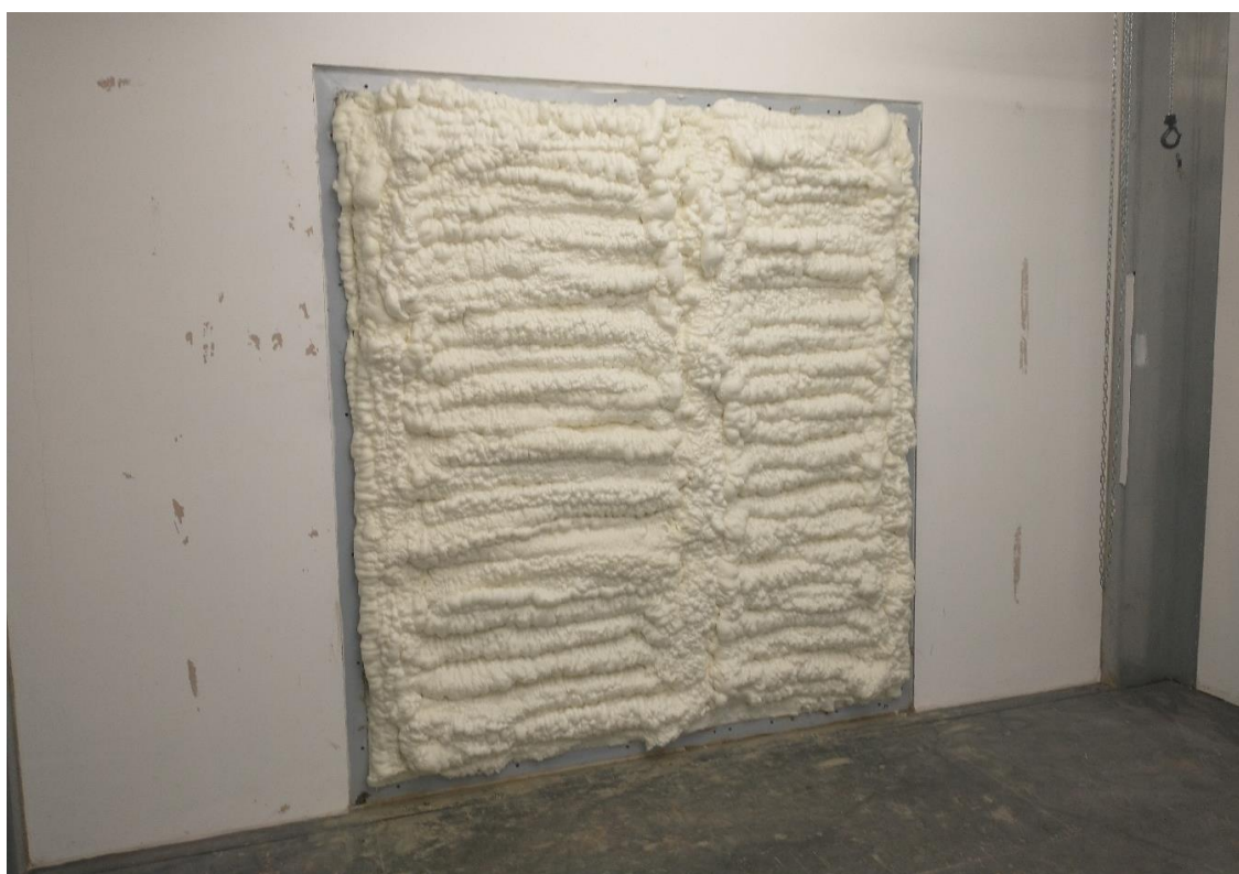
Figure 5.2- Photograph of spray foam applied 100 mm, first application
